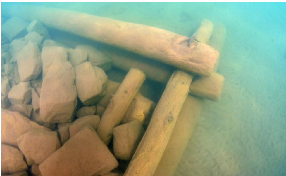
Figure 41. Hermit Island north crib construction detail
