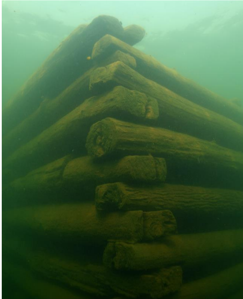
Figure 28. Bass Island Quarry's main crib corner system
