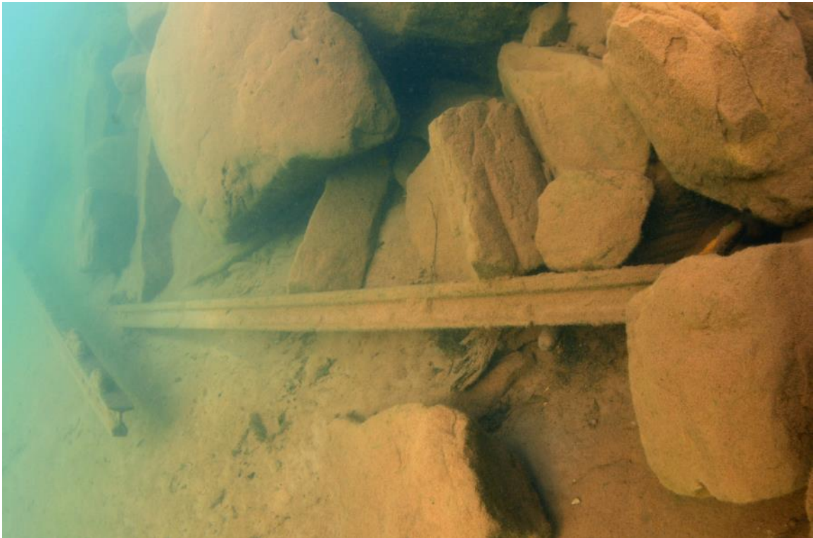
Figure 44. Rail track segments
